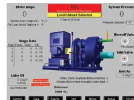
At left is an example of HMI screen displays we develop for control systems. This one is for a compressor.
