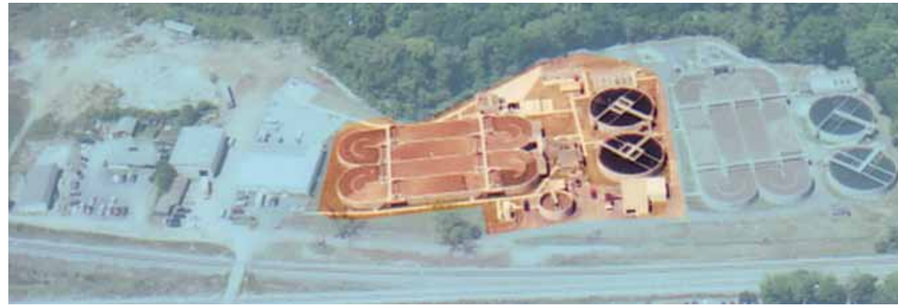
Aerial view of the Alabaster wastewater treatment plant with the expansion portion of the plant highlighted (center).
