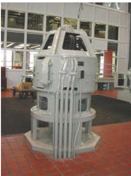
One of the older DC motors in the pump station building. Revere's equipment is installed in the room in the rear of the photo.
