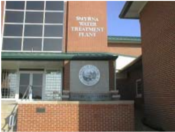
Filter building entrance
