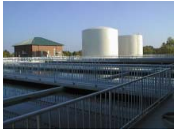
Settling basins, chemical feed building, and tanks
