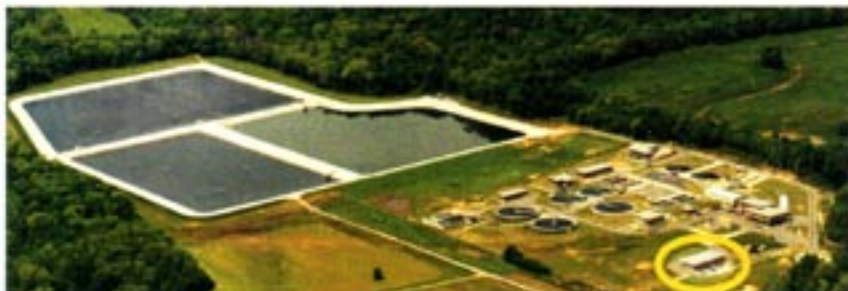
Influent pump building (highlighted) is located in lower right of this aerial view of the plant.
