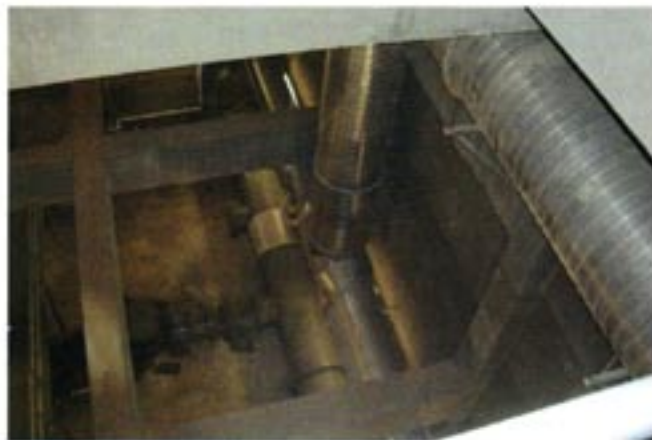
Looking down into a dry well from the ground level floor.
