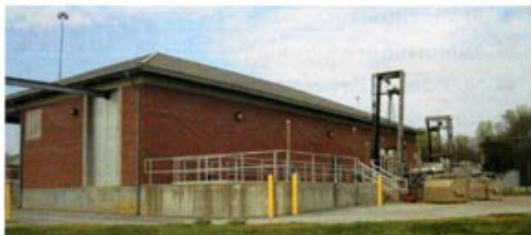
Exterior of the influent pump building showing wet wells and rakes (at right of building).
